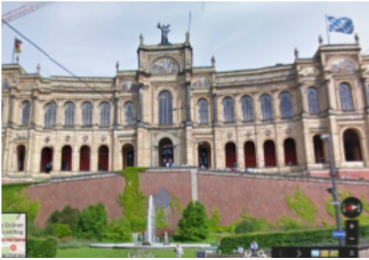
Figure 52: State parliament ( Landtag ) in 2008, seen from the west (Bavarian flag above the south wing).
