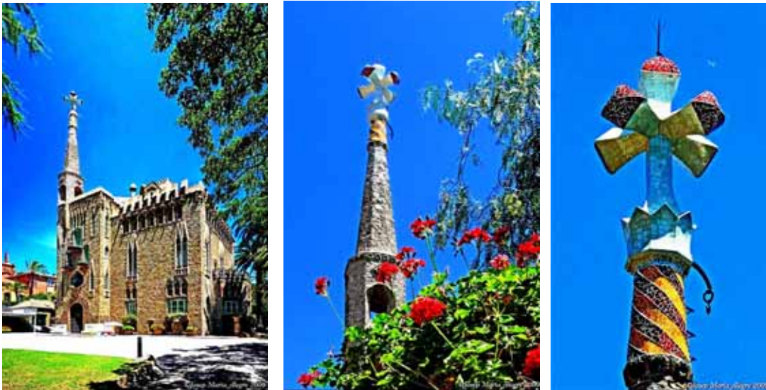
[38] Torre de Bellesguard (1900–1909)
