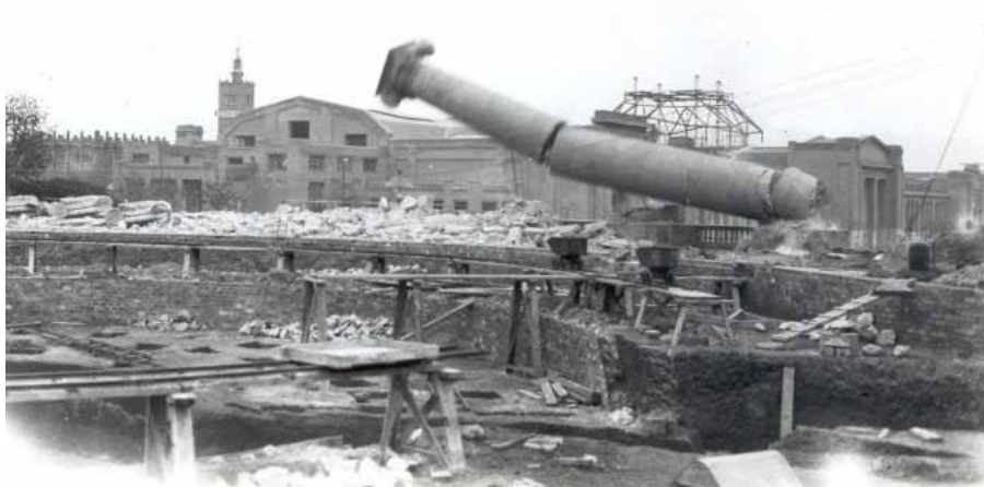
[104] Columns coming down (1928)
